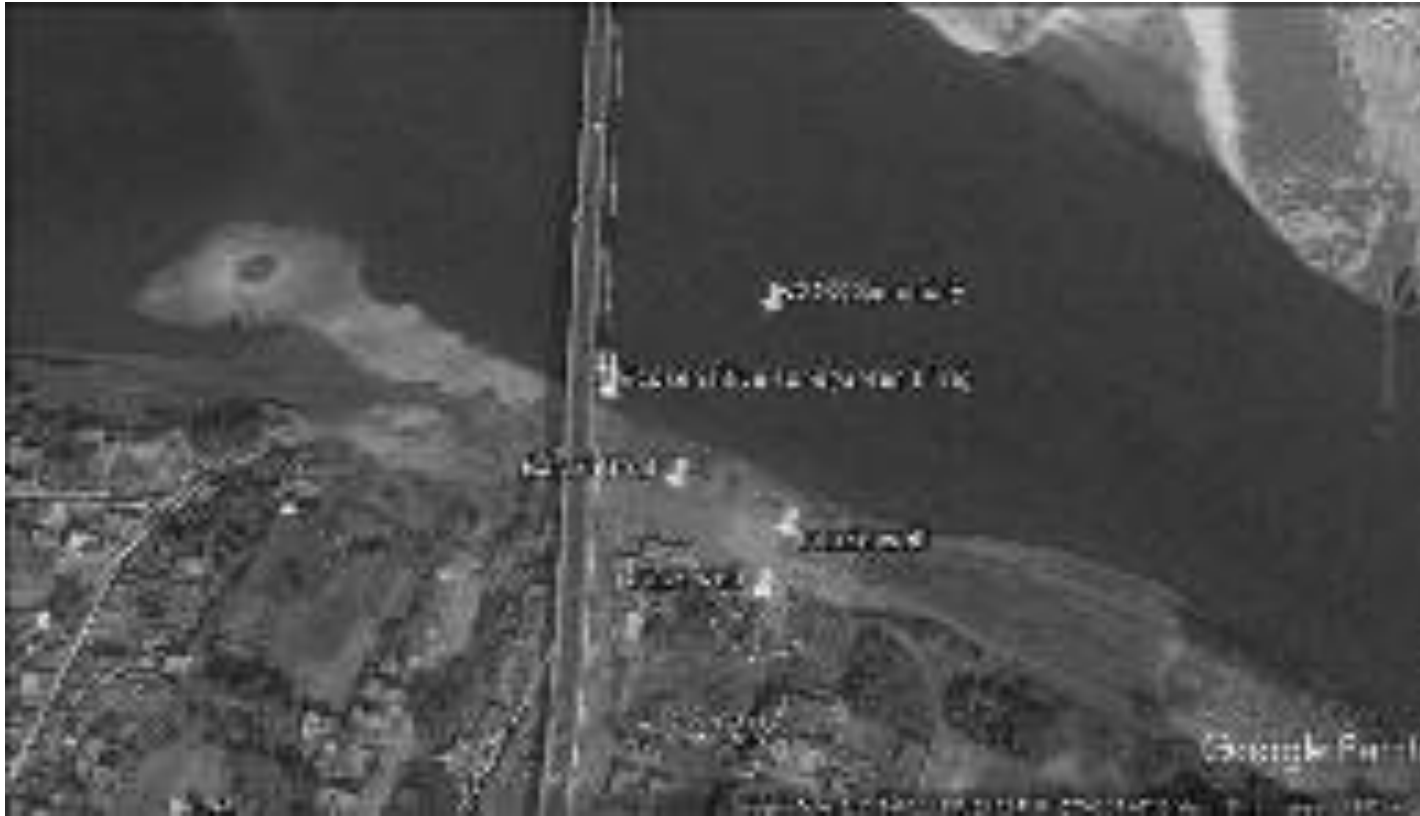
Figure 12: Eco sensitive zone, Vikramshila Gangetic Dolphin Sanctuary (VGDS) and intake structure
