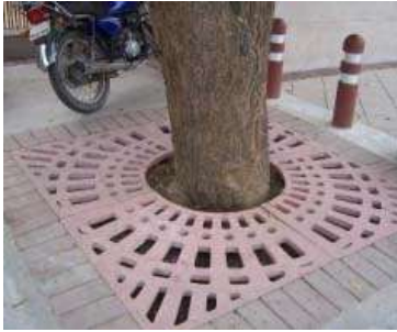
Figure 8-6: Example of RCC tree guard to prevent soil erosion
