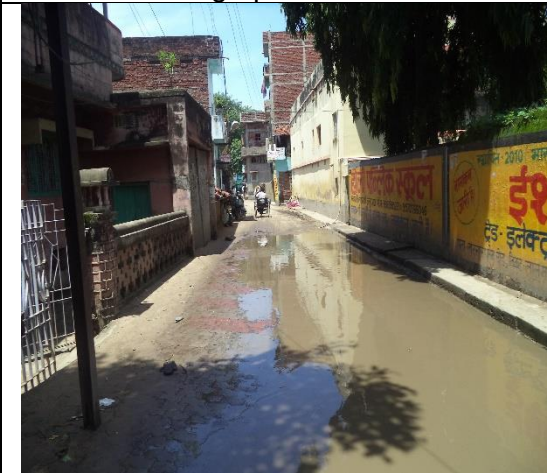
Location Photograph - 3 Rising Main to Delha
