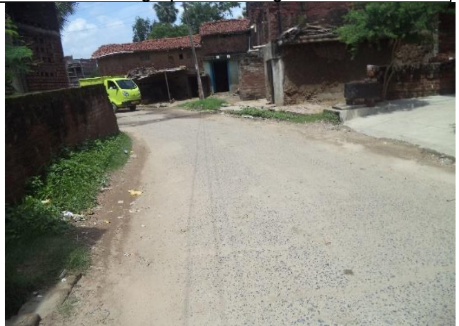
Location Photograph - 4 Rising Main to Delha
