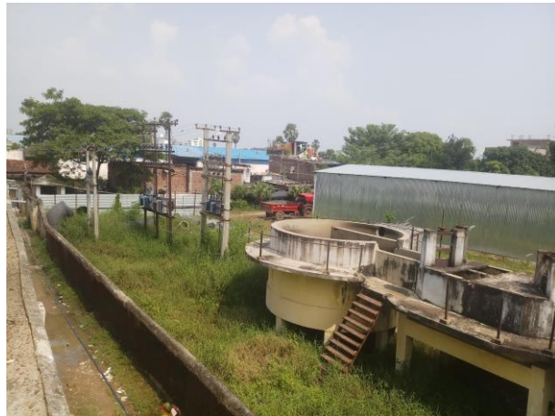
Existing STP at Pahari
