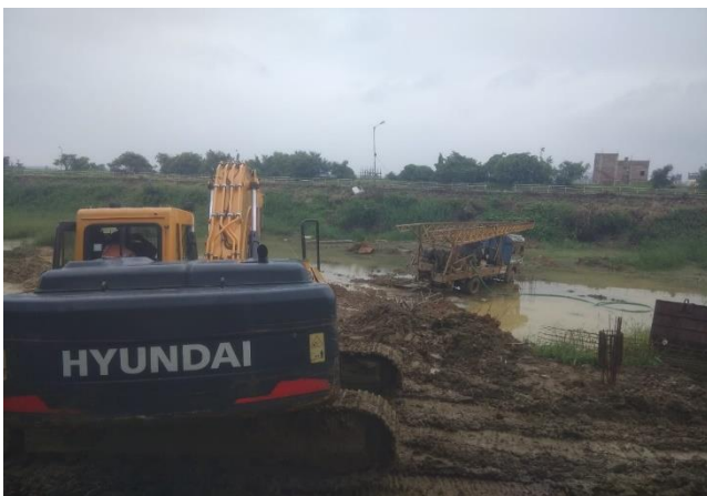
Construction work – Pahari STP
