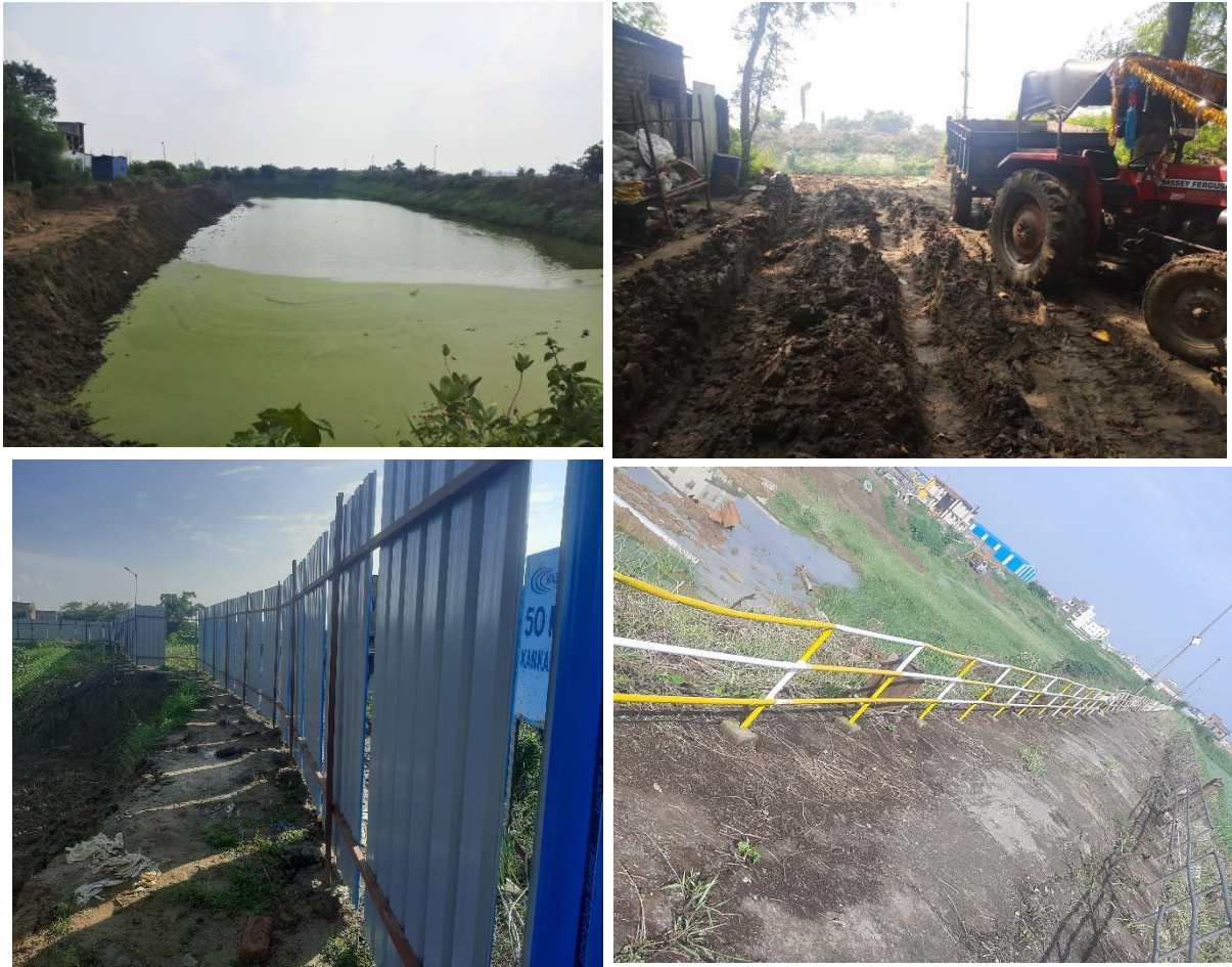
Construction work – Kankarbagh STP
