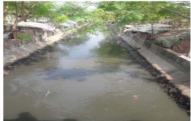
Figure 2: Main Drain at Kankarbagh zone-Yogipur drain
